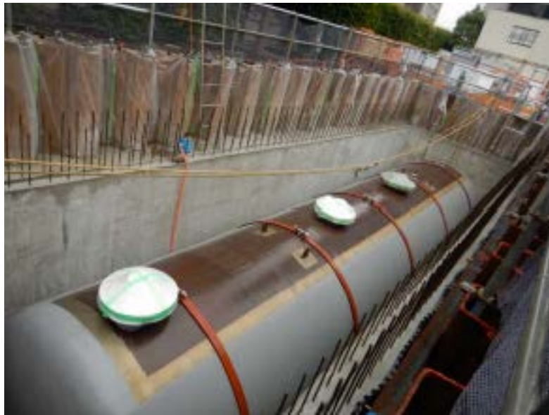
Emergency oil tanks during construction (photograph June 2020)
