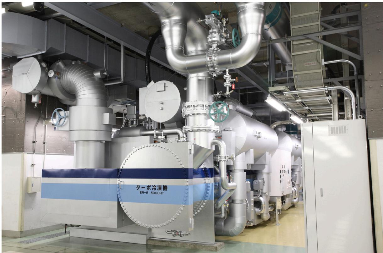
*Photo: The new 5,000-refrigeration-ton electric turbo chiller*
